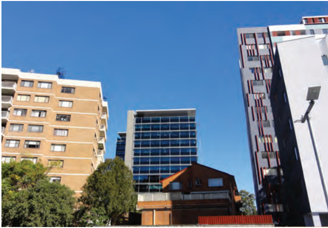
3 storey walk up building between taller element on the western boundary with a 13 storey commercial building behind facing Charles Street
