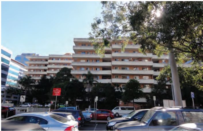
9 storey residential building to the north of the subject site on Macquarie Street
