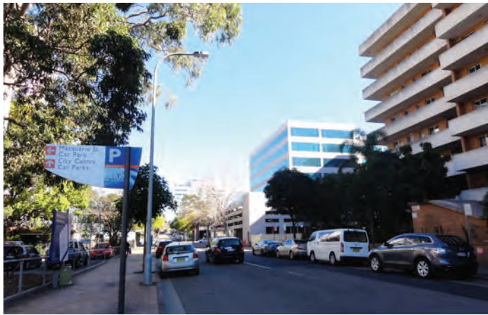
Macquarie Street streetscape and built form - view from east - subject site on the left
