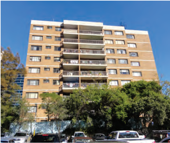
9 storey residential building on the south-western corner of the site
