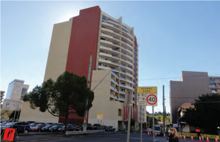
26-30 Hassall Street - 17 storey building to the east of subject site presenting a blank wall toward the site
