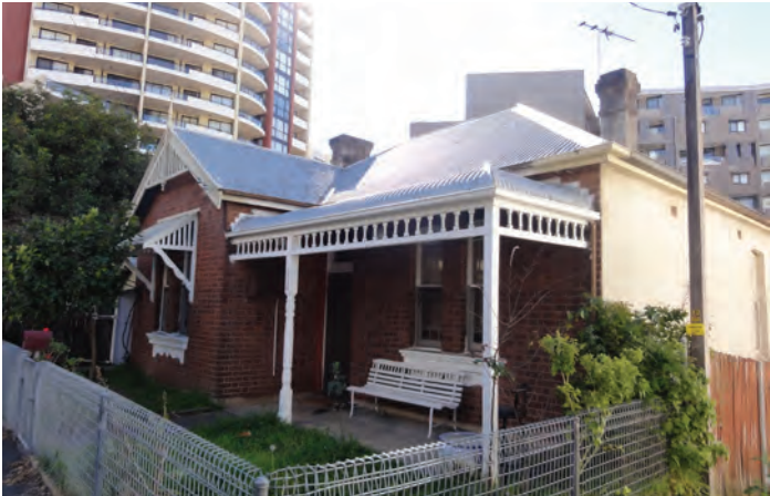
Heritage cottage on Wigram Street
